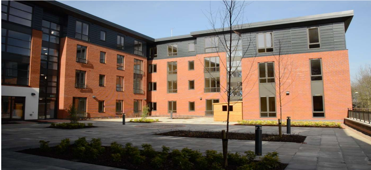
Parklands View, an Extra Care facility in Darley, Derby
