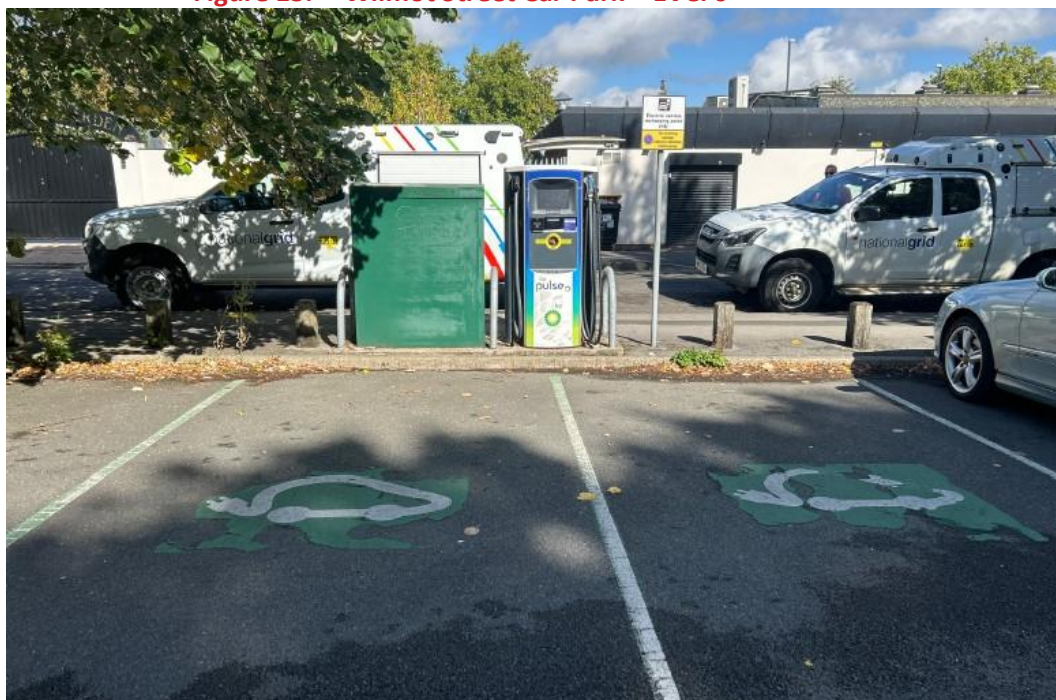
Figure 15. Wilmot Street Car Park – EVCPs
