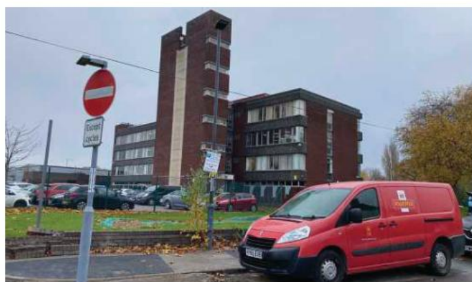
Top: the Royal Mail sorting office is out of scale to the other buildings along Midland Road
