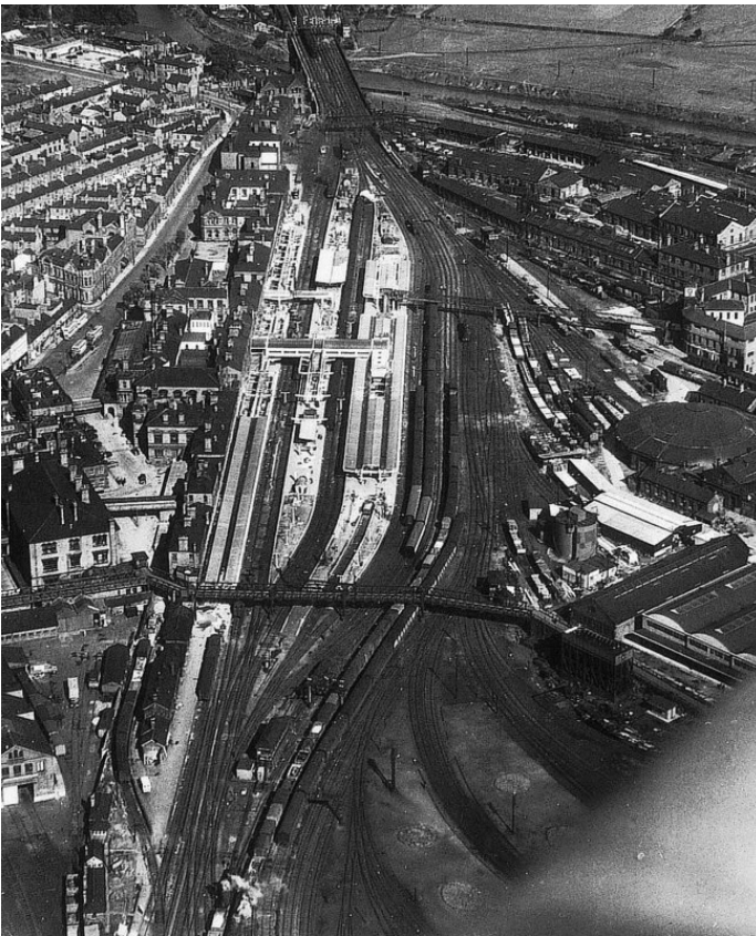
Historic aerial photograph showing the construction of the previous individual platform canopies, that replaced the earlier enclosed train shed.
