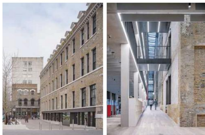
Restoration and extension of a Grade II Listed former hospital building – Tower Hamlets Town Hall
