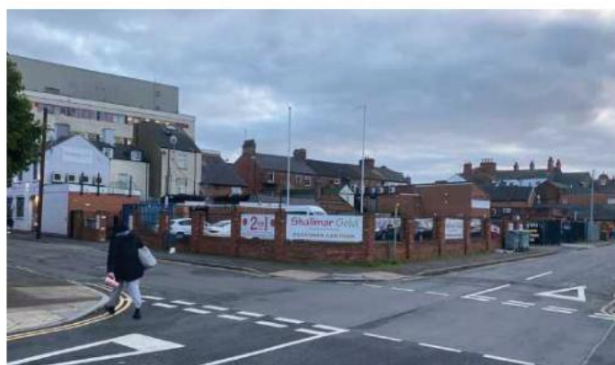
Top: Mixed quality retail units fronting Midland Road Bottom: The Wellington Street frontages have been cleared, and the rear of the block is used for surface level car parking
