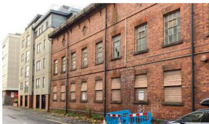
Top: The buildings immediately outside the station entrance form a cohesive and well-preserved historic cluster
