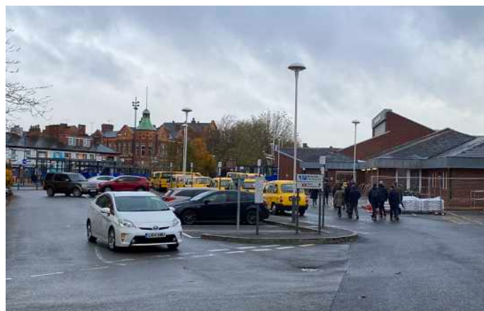
No sense of arrival at the principal, western station entrance
