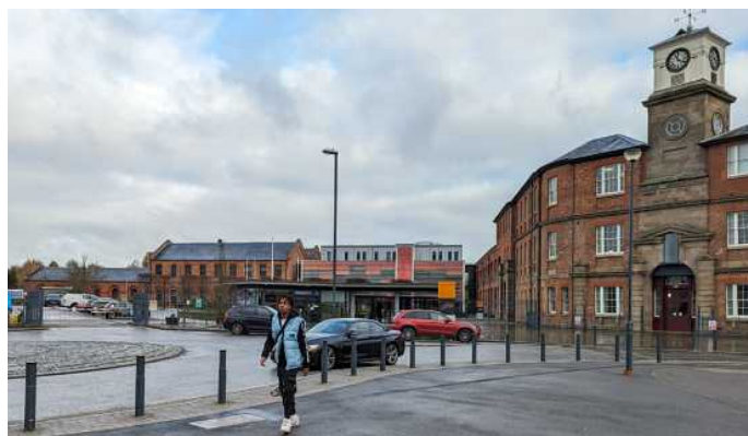
Images from top: Former railway workers houses on Calvert Street; Retail units fronting Railway Terrace; St Andrews House, a rehabilitation centre on London Road; and Derby College, including a cluster of Grade II and Grade II* Listed buildings
