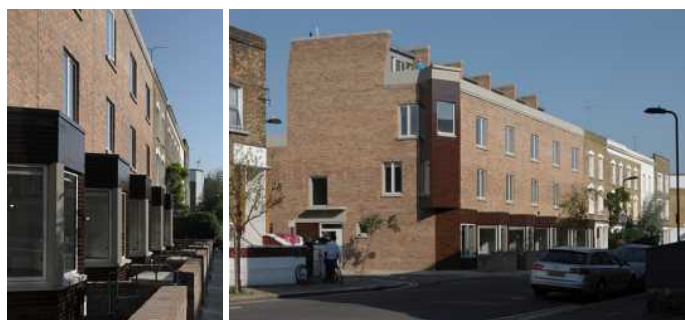
A row of terraced houses completes a bomb damaged urban block – Aikin Terrace, London
