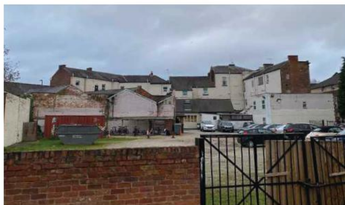
Top: The unattractive shop units fronting Railway Terrace Bottom: The rear of the block has been cleared, and is used for surface car parking
