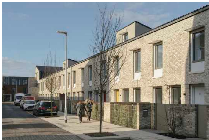
Medium density, affordable housing development, a modern take on railway workers housing – Goldsmith Street, Norwich
