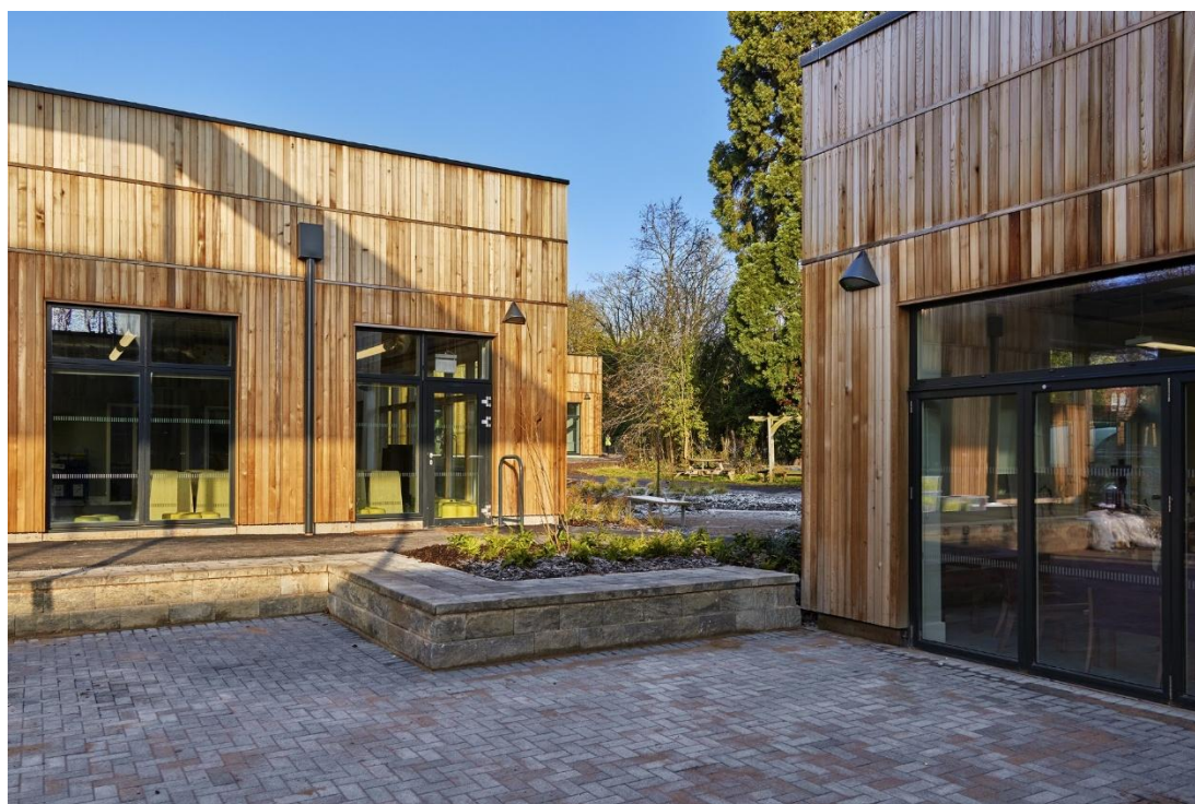
Figure 48: Chapel Courtyard, St. Mary's Catholic Voluntary Academy
