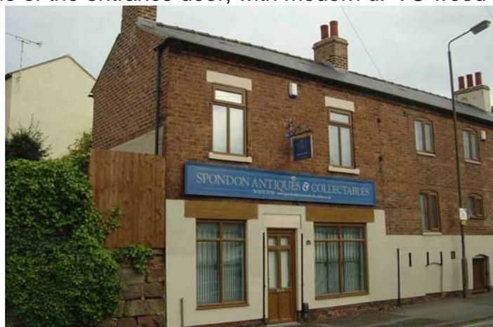
area, with one bricked up. The first and second floors have six modern casement windows within the original window openings with brick relieving arches, apart from the first floor central window which has had the sill height lifted.
