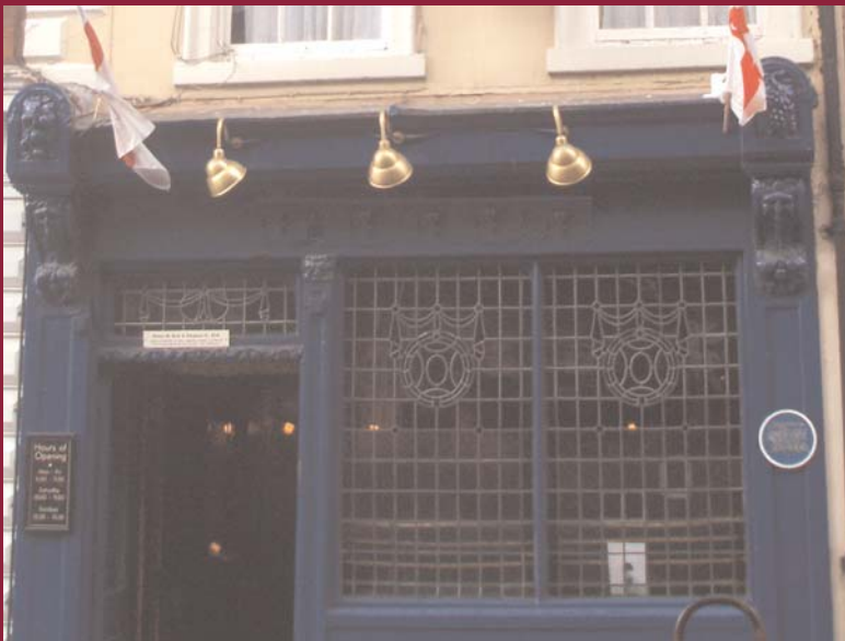
unacceptable fascia illumination
