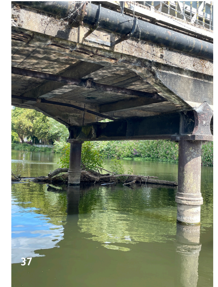
37. View looking at Pier 3 (8.8.25).
