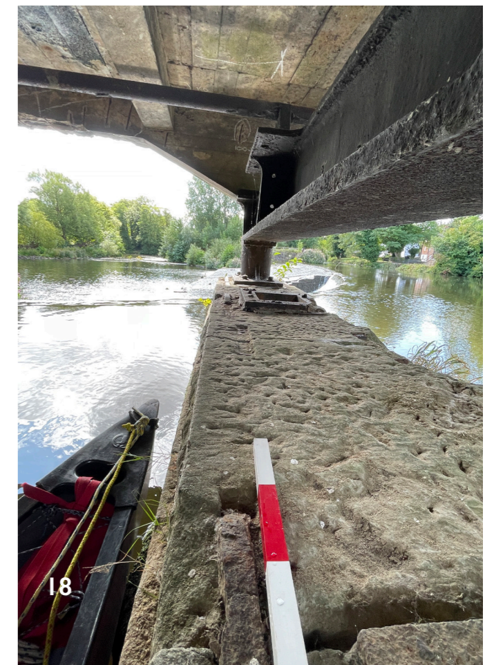
18. Masonry upper face to Pier I (8.8.25).
