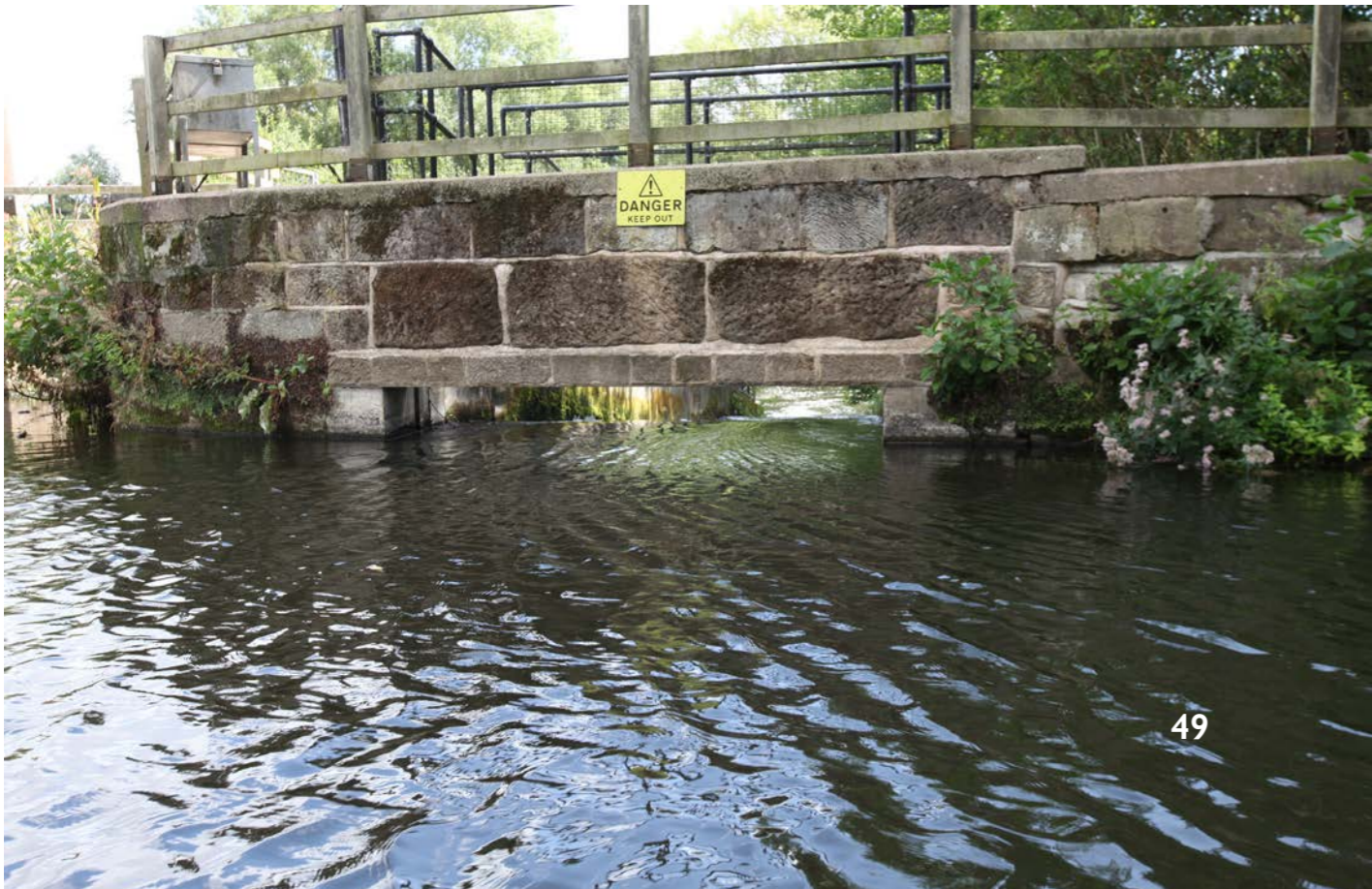
Mel Morris Conservation - Darley Abbey Bridge
