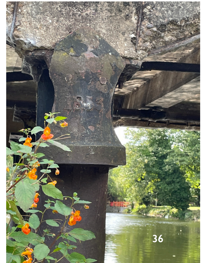
36. Casting with 1853 date - upstream (pier 3) - 8.8.25
