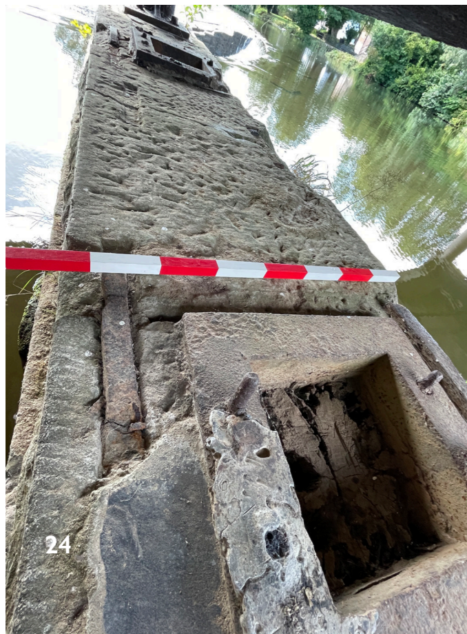
24. Casting to former post (upstream) - 8.8.25.
